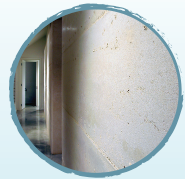
Rammed limestone internal walls
