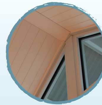
Timber V groove lining
